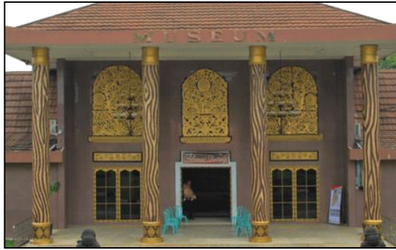
Gambar 5 : Foto Pillar Museum Balaputra Dewa Sumber: Ferry Muhammad Rahman, 2023
